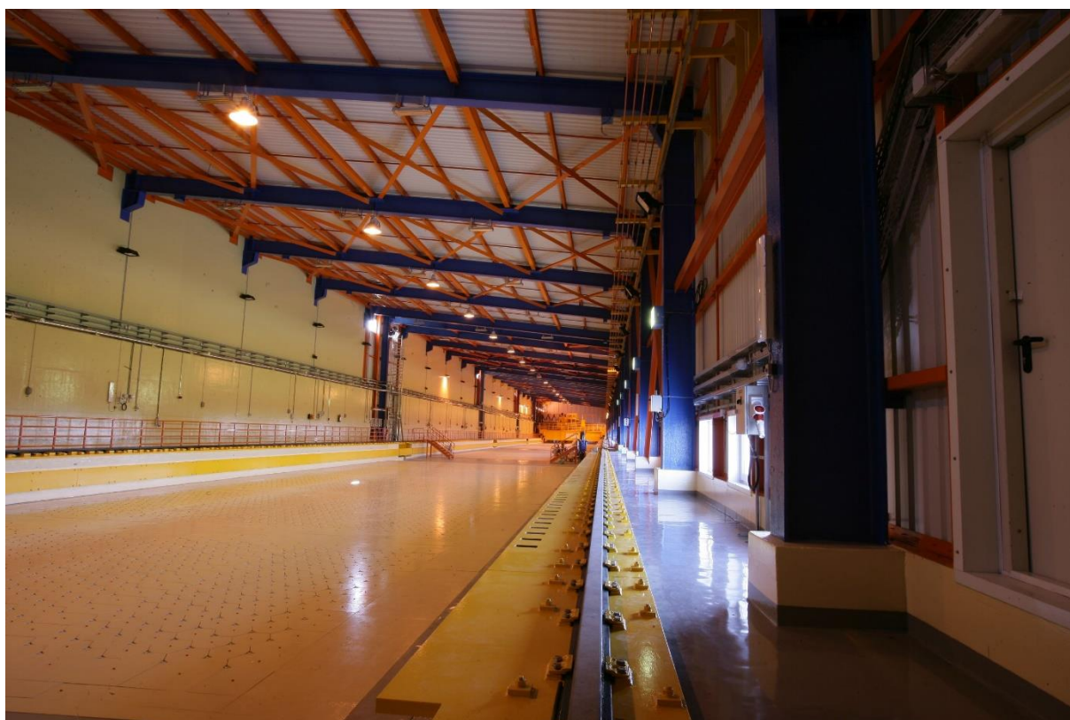
Figure 1 Loading hall of the SFISF (source: http://www.rhk.hu/ )
